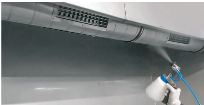
Ventilation systems: For the targeted disinfection of the air inlet you will find the nozzle for the larger throw range in the scope of delivery.
